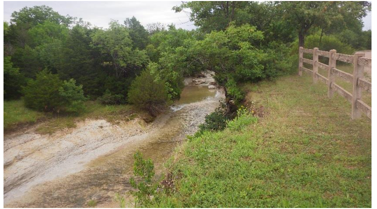
Photograph 6 - Overview of APE, view to the east.
