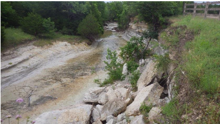
Photograph 7 - Overview of APE, view to the east.
