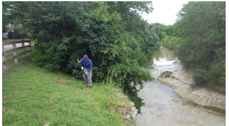
Photograph 8 - Excavation of ST 04, view to the west.
