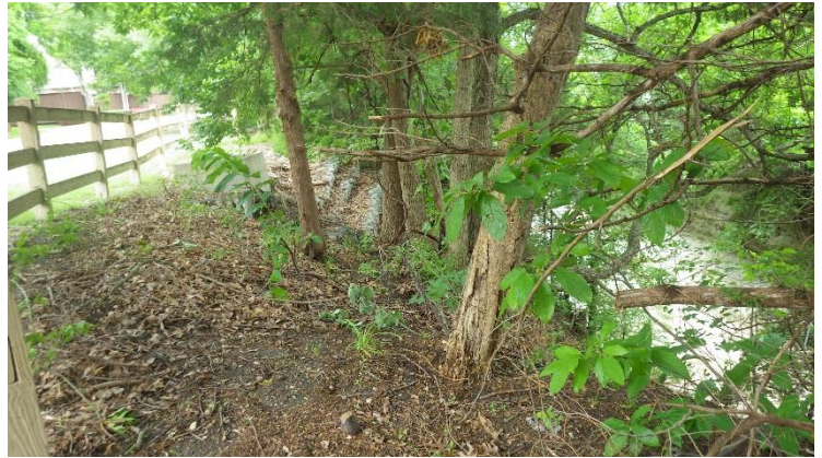
Photograph 28 – Rock rip-rap retaining wall, view to the west.
