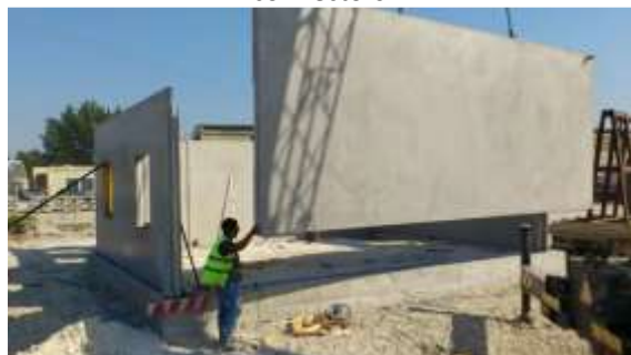
Figure 9 - Installation of the sandwich panels.
