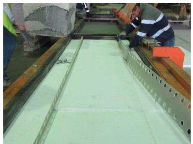
Figure 6 - Application of the EPS insulation core material and continuous GFRP connectors.
