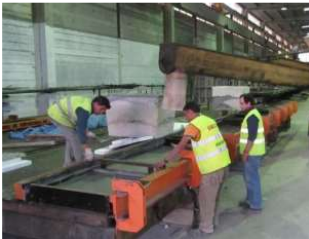
Figure 5 - Casting the bottom SFRSCC layer.
