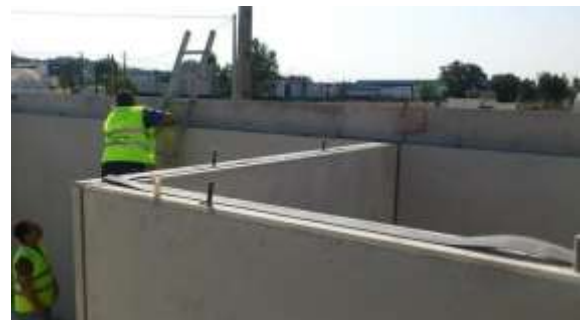
Figure 9 - Installation of the sandwich panels.
