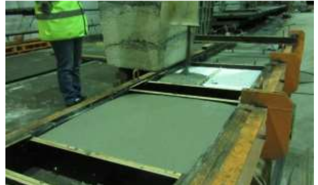
Figure 8 - Casting the top SFRSCC layer.
