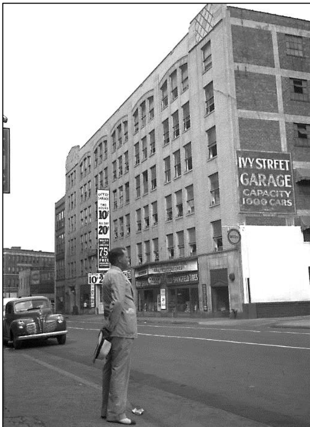
Figure 26. Ivy Street Garage, October 27, 1946.
