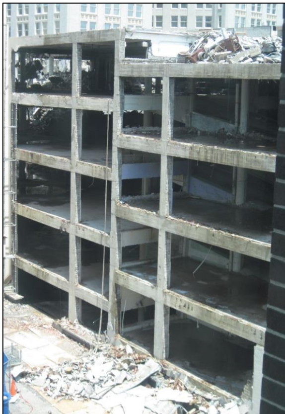
Figure 27. Kell Hall being demolished, August 3, 2019.
