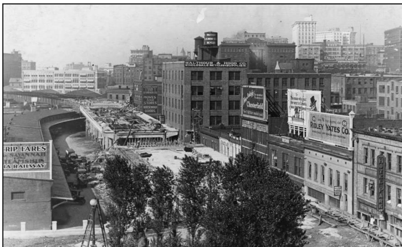
Figure 8. Spring Street viaduct under construction, 1923.
