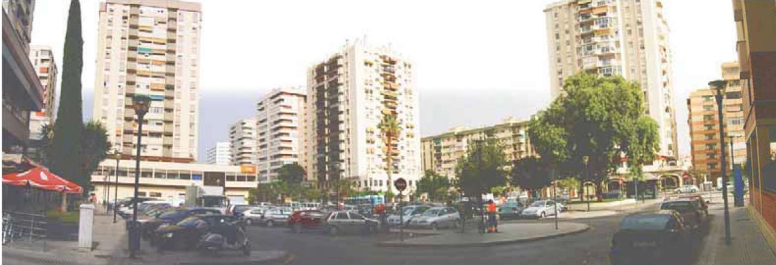
Fig. 1. View of the parking area in the study case. Source: by authors
