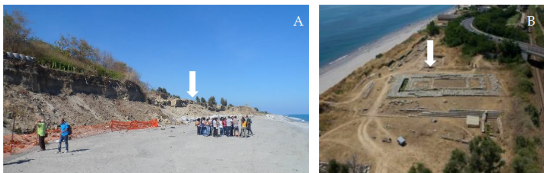
Figure 2.40 (A) Damages caused by high waves during 2015 at Monasterace Marina (Ionian south coast of Italy); (B) Hellenic archeological site ( IV century BC) protected by the structure is individuated by the white arrow; image source: www.bivongitheristis.altervista .
