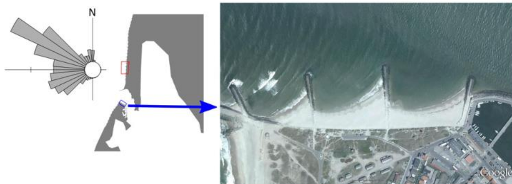
Figure 2.21 Example of a Groyne field where the shoreline in the left side is turned against the prevailing wave direction; the latter can be deduced from the rose diagram on the right side of the image (Kristensen et al., 2016).
