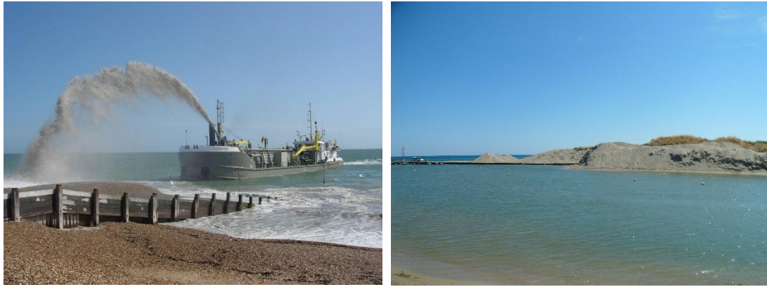
Figure 2.35 (A) Dredge during a beach replenishment in UK, image source: www.escp.org.uk/beach-nourishment ; (B) Dredged material at the harbor mouth at Laghi di Sibari, Crati river's mouth (Calabria, South of Italy).
