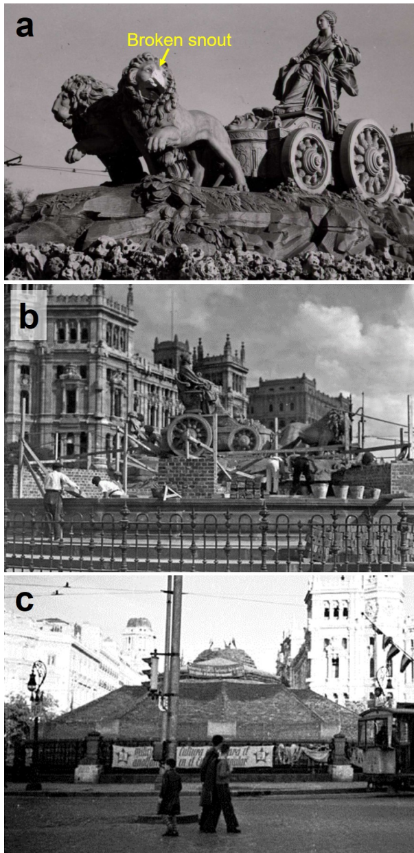
Figure 7. Fuente de Cibeles during the Spanish Civil War. a: Photograph, 1936. Lion with damaged snout; b: Photograph, 1937. Fuente de Cibeles began to be covered under a pyramid of sandbags and bricks on July 3th, 1937; c: Photograph, between 1937 and 1939. Protected Fuente de Cibeles
