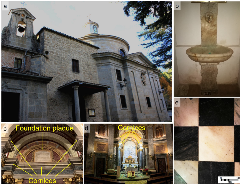
Figure 12. Santuario de San Pedro de Alcántara . a: West facade of the Sanctuary, on the right side the Royal Chapel can be observed, b: Basin carved with Montesclaros marble in the sacristy; c: Interior of the Royal Chapel where the founding plaque and cornices sculpted in Montesclaros marble can be seen; d: Interior of the Royal Chapel, cornices carved in marble from Montesclaros; e: Paving of the Royal Chapel, the white slabs are made with Montesclaros marble.
