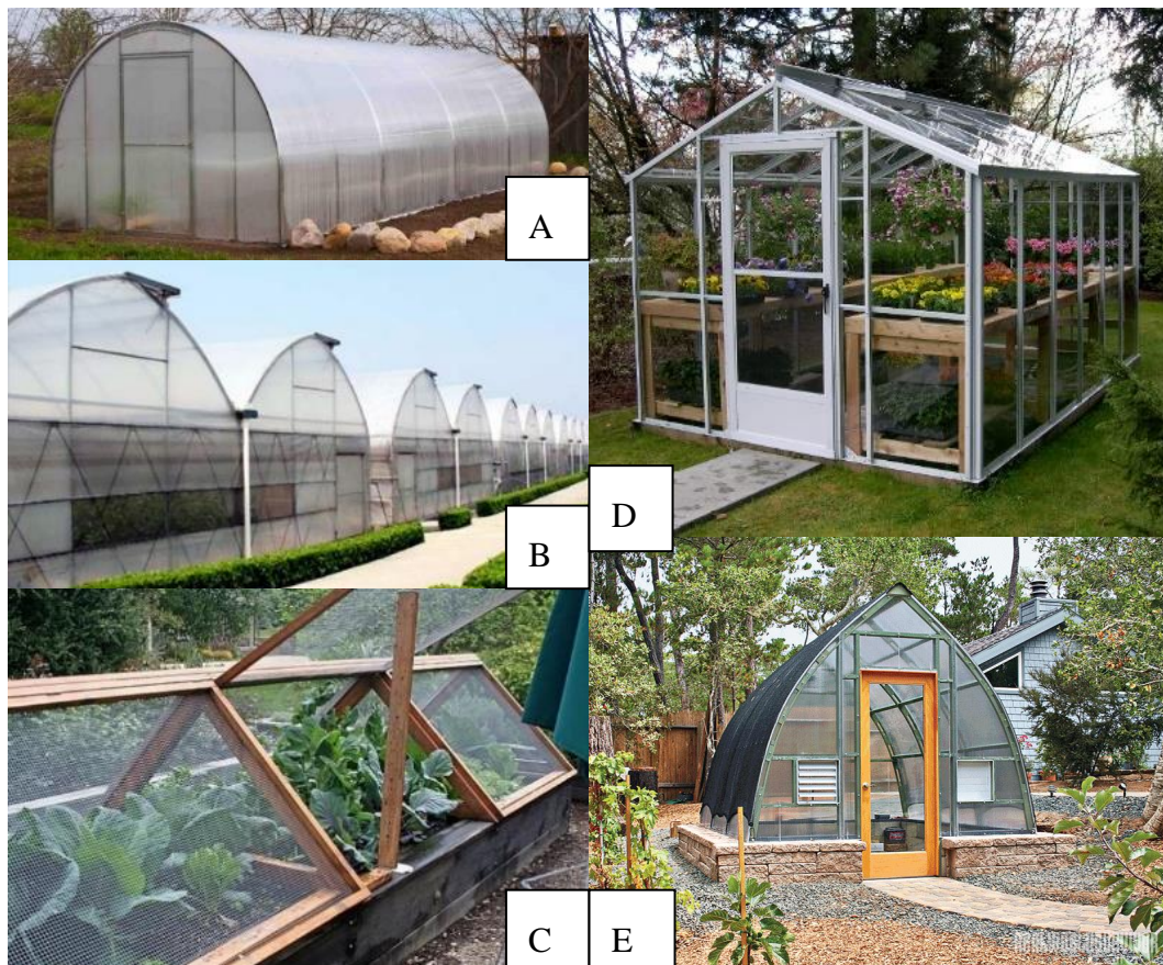
Figure 2.40 Single pan greenhouses. A) Hoop. B) Arch roof. C) Cold frame. D) Gable roof. E) Gothic [61-65].
