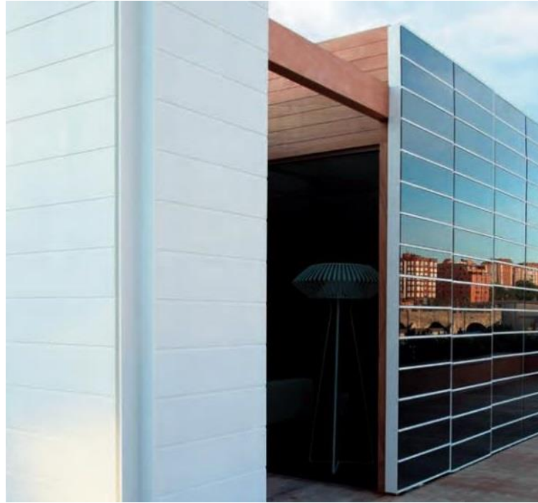
Figure 4.5 Corian® pre-fabricated ventilated façade with Onyx Solar PV glass [83].
