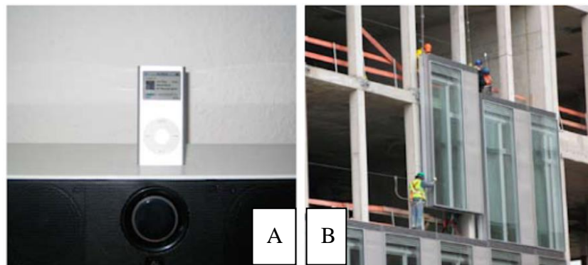
Figure 4.1 The plug & play concept. A) On portable music player. B) On curtain walls.
