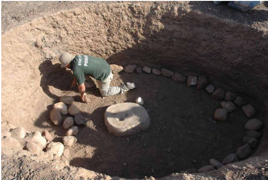
Figure 9 Laying of the foundation layer of boulders.
