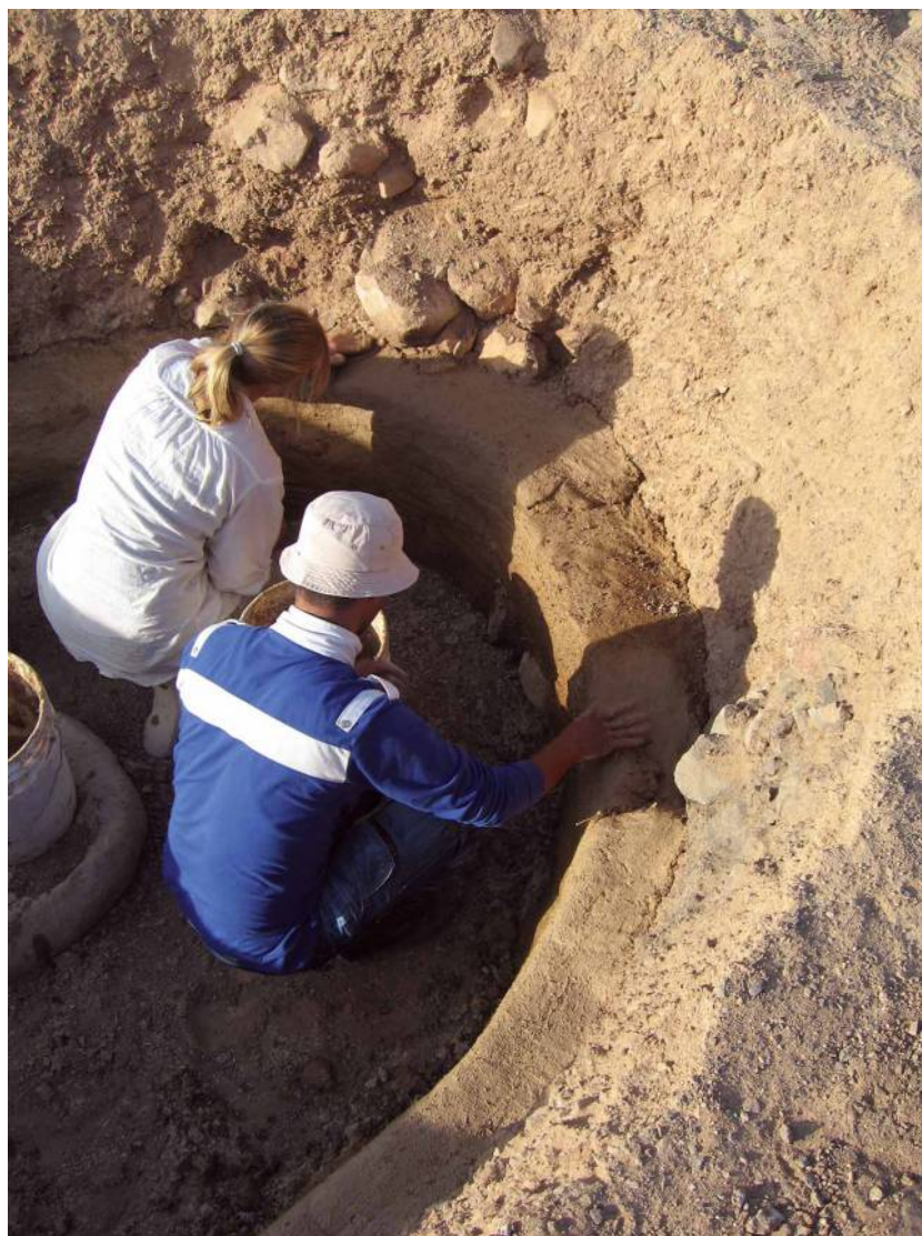
Figure 10 Application of wet pisé layers of 10–15 cm thick each.
