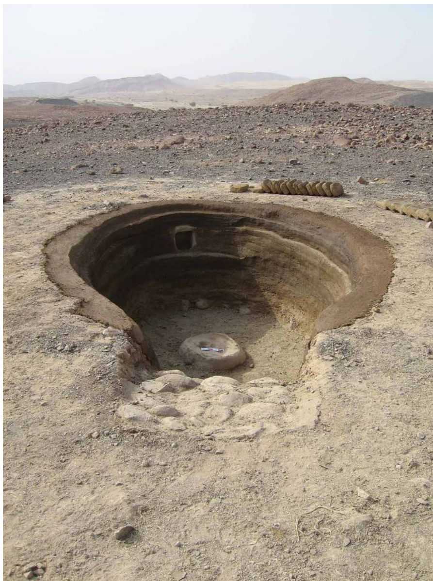
Figure 12 The finished pisé wall (looking north-west), with the ramp on the foreground, and the niche in the west part of the wall. The different layers are drying in different colours. The stepping in of the wall is visible.
