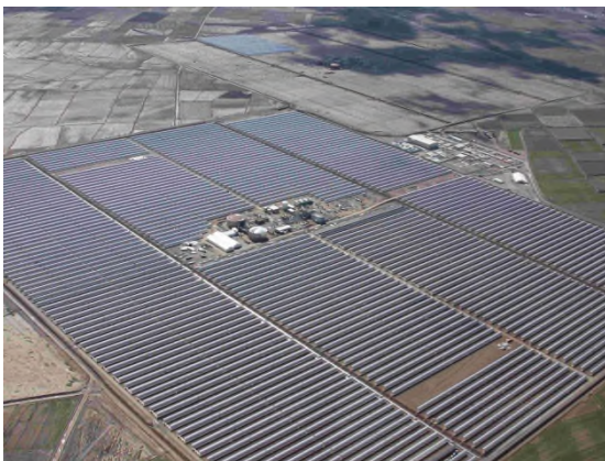
Figure 2.2 - AndaSol plant in Spain
