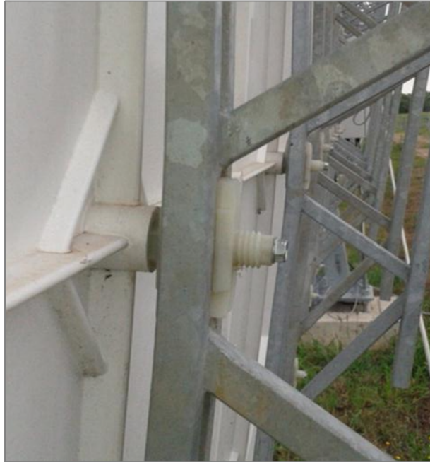
Figure 4.52 - Ronda mirror support adjustment
