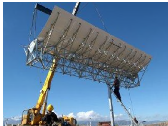
Figure 2.3 - Large parabolic trough and support structure
