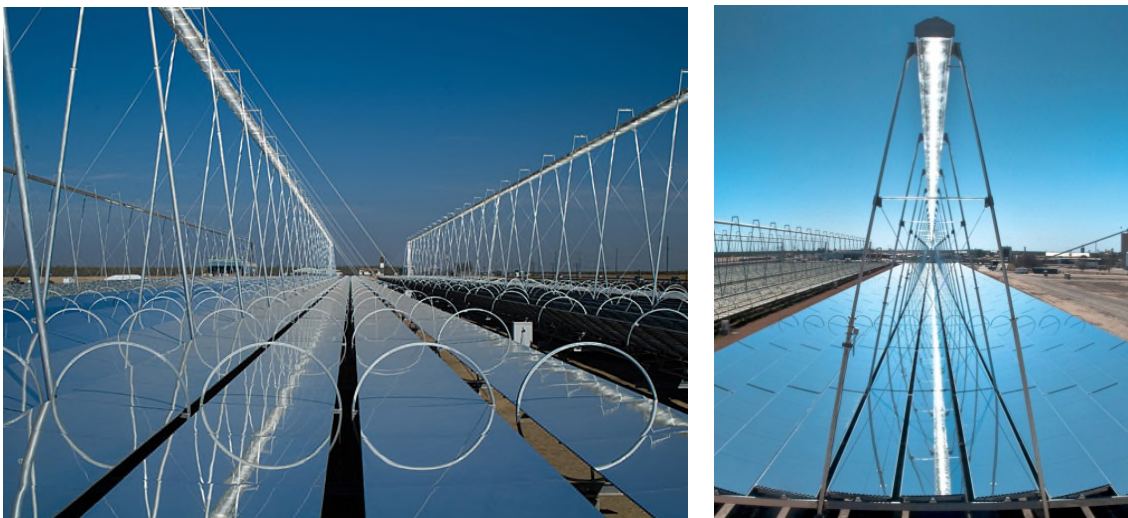
Figure 2.5 - Areva Solar Linear Fresnel collectors
