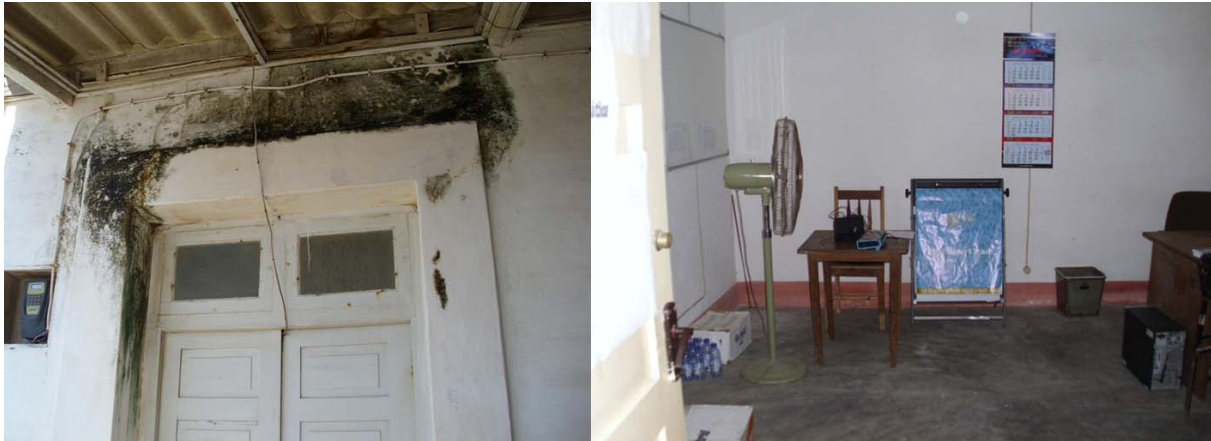
Figures 5 and 6 – Examples of Photo 02. They portray: 4. The external walls of the CMC of Ilha de Moçambique; 5. Missing equipment, again in Ilha de Moçambique.
