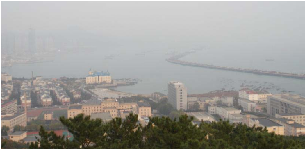
Photo 14: The uncompleted Dalian Xinghai Bay Cross-sea Bridge (Pulandian Bay Bridge). It is said to be the biggest continuous beam sea-crossing bridge in Northeast China and replaces the congested coastal road.
