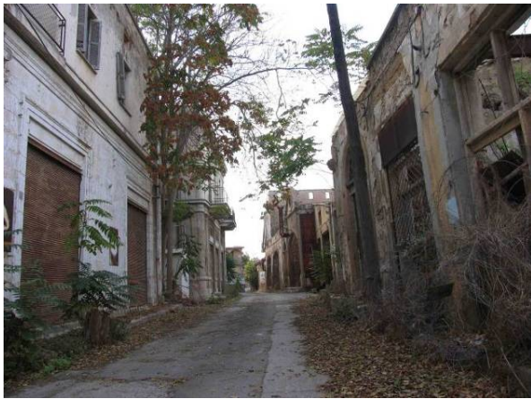
Figure 1: A view of a street in the buffer zone
