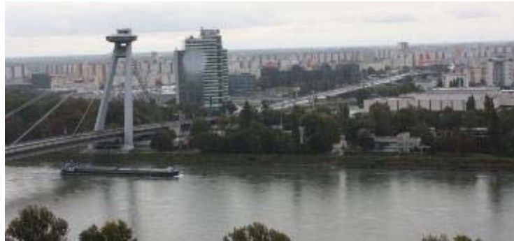
Figure 8: Petržalka – structures of large housing estate from Bratislava castle (photo by author).
