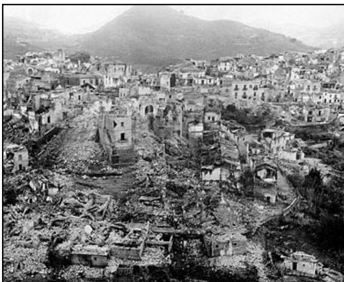
Figure 3.4: Belice – post earthquake in 1968
