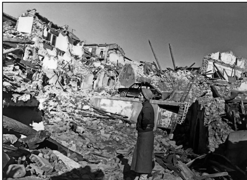
Figure 3.6: Disillusioned woman gazes at the impacts caused by the Irpinia earthquake
