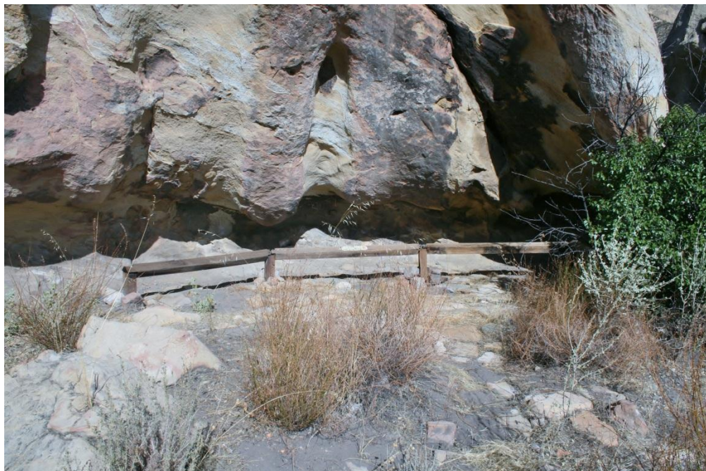
Figure 9.2: Photo of the main shelter at Condor Cave taken by Michelle L. Wienhold on October 2011.
