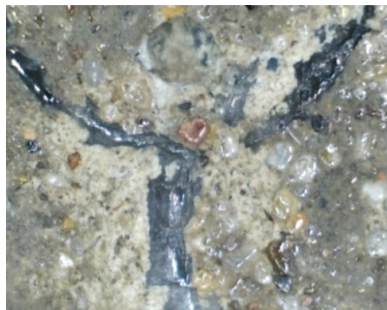
Figure 5. Large cracks (>1mm) filled with mineral crystals in adversely cured concrete.
