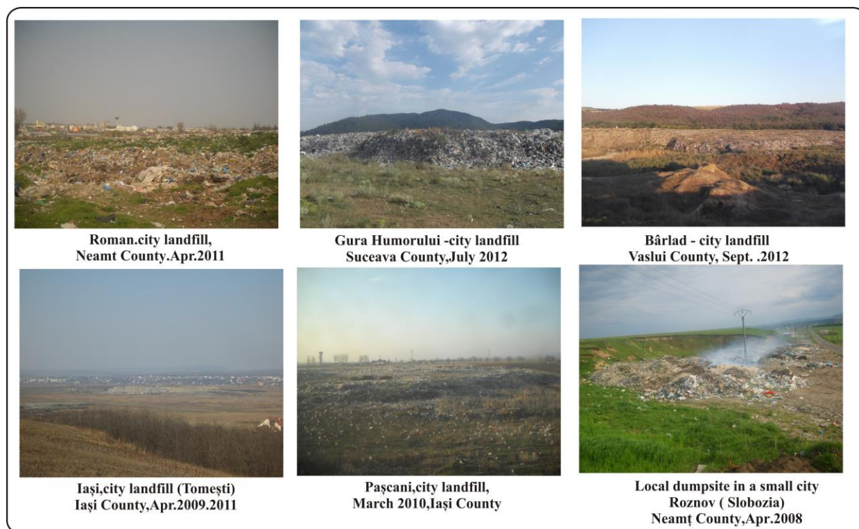
Figure 3: Non-compliant landfills from study area
