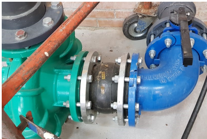
Figure 4.2: Current tube and flexible joint.
