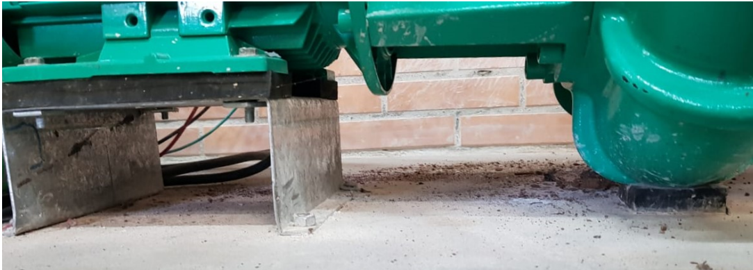
Figure 4.1: Current centrifugal water pump foundation.
