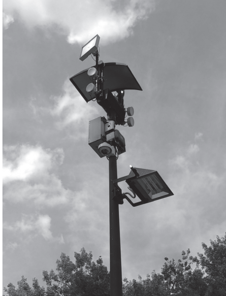
Figure 5.2: Video camera, sound sensors, special lighting technology, wifi tracking technology and possibly other surveillance technologies in front of the Sint-Catharinakerk close to the main entrance to the Stratumseind street (photo taken by author, 26 August 2018)
