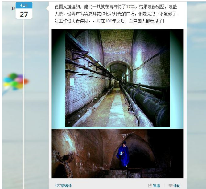
Figure 6.5 The German-built sewage system in Qingdao
