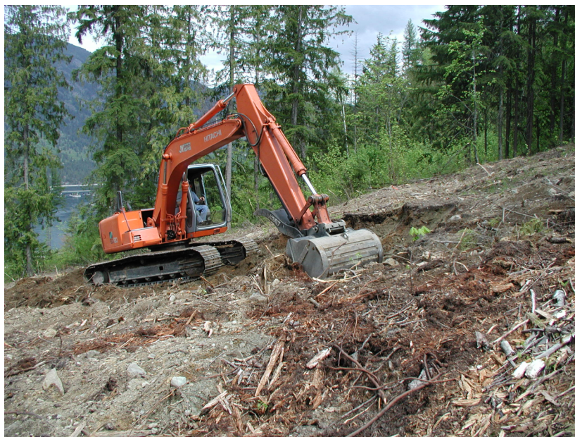
Raw Land Prior to Garden Construction
