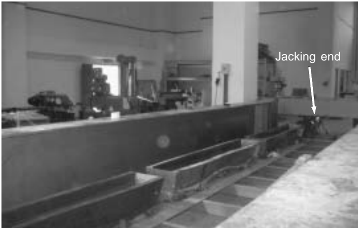
Plate 1: Arrangement of Sleeper Moulds on Stress Bench
