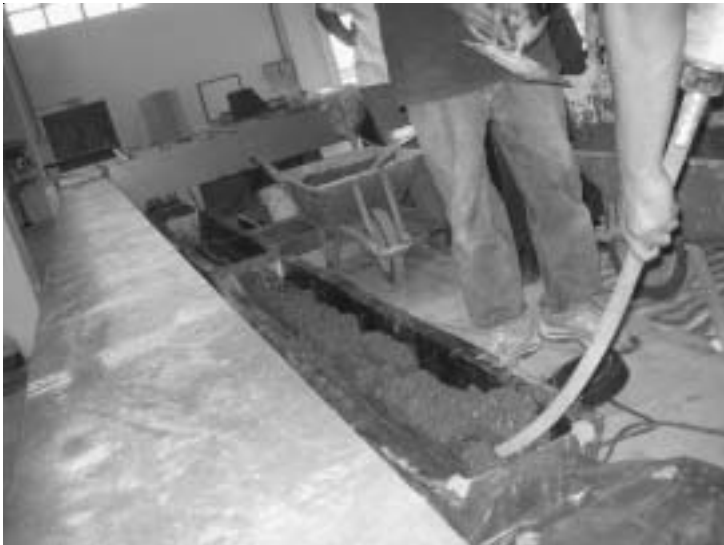
Plate 2: Concrete Placement in Moulds
