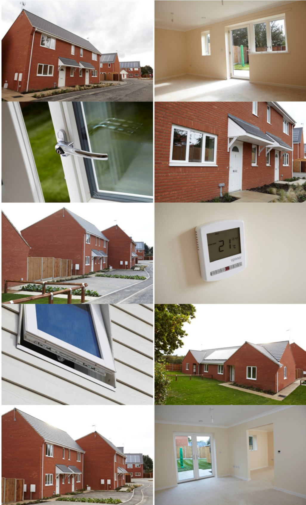
Figure 3.2 – Photographs of Trinity Close, Rackheath
