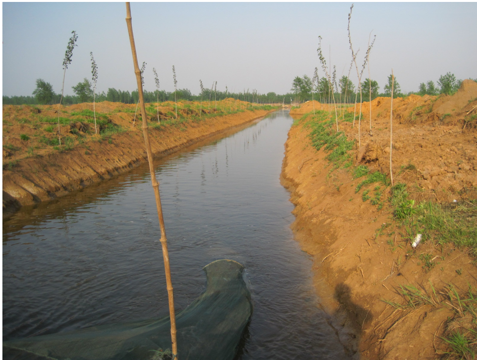
Figure 5-10: A recently widened drainage ditch in Wanzhuang.
