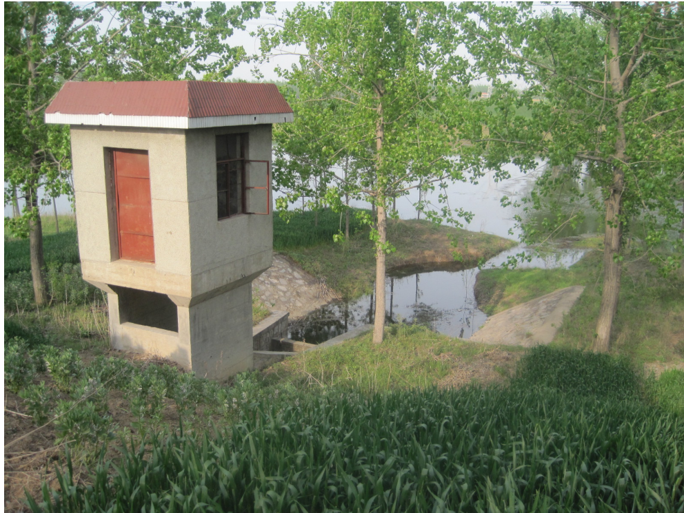
Figure 5-11: A drainage gate to manage floodwaters in Dongdian.
