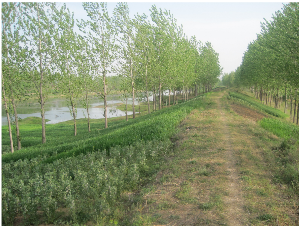
Figure 5-12: The levee protecting Dongdian from the FeiHe River.
