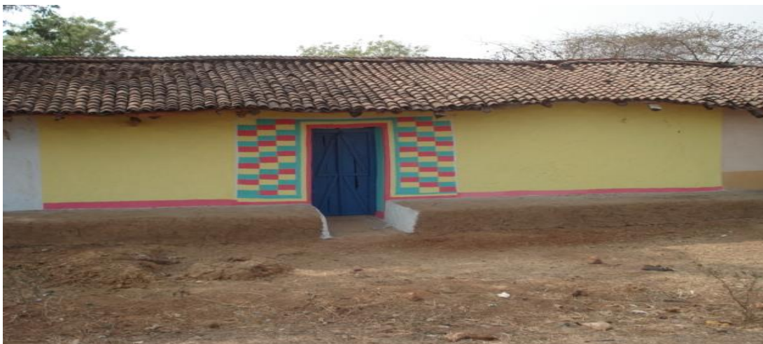
Photo 3-2: A freshly painted Chhattisgarhi house
