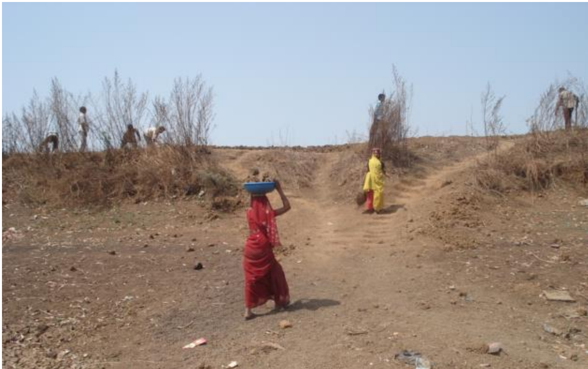
Photo 7-3: Women carry away earth from up the pond slope and deposit it over the edge
