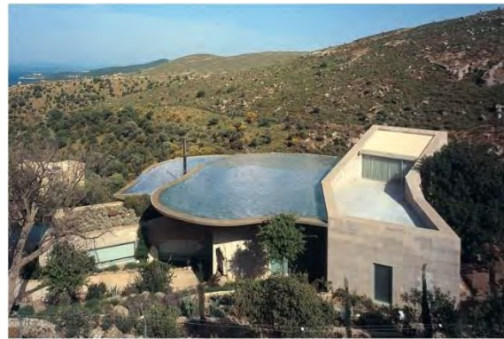
Figure 3.3 – Roof pond system [20]
