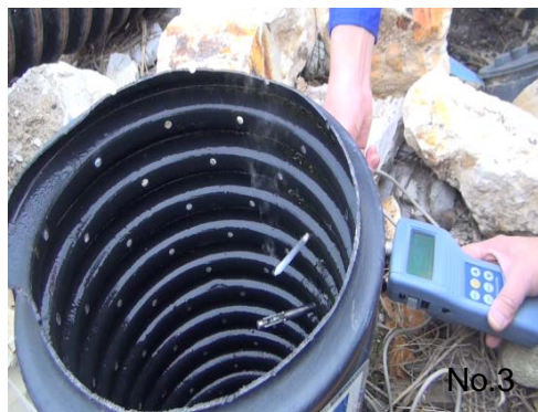
(a) Outflow vent (No.3)
