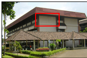
(a) RC building with brick masonry infill
