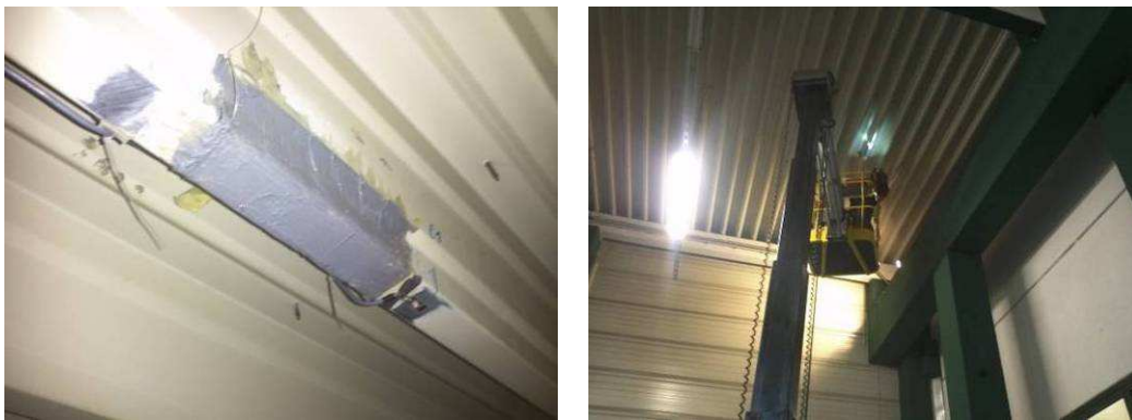
Figure 7: Laminated GFRP sensor and installation at the roof construction.
