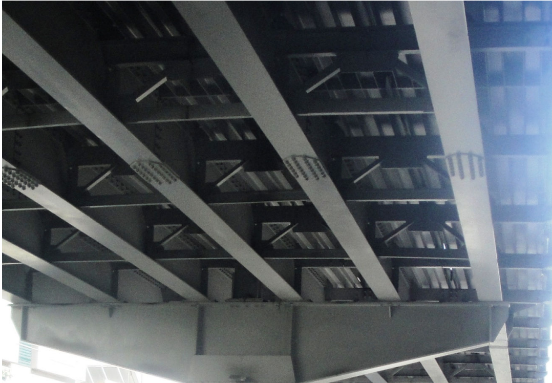
Figure 2: The lateral trusses connecting the deck girders together
