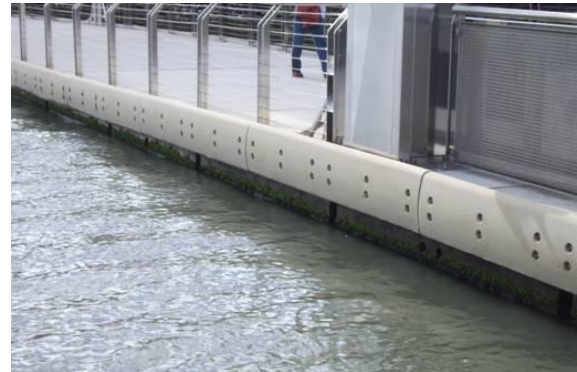
Figure 5: Fibre composite reinforced waler
