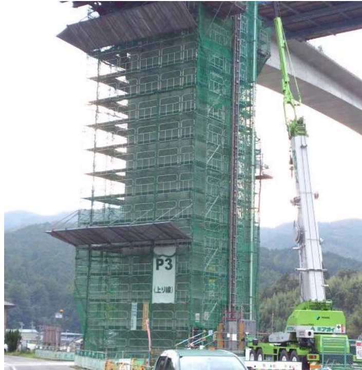
Figure 1: Prefabricated scaffolds assembled by Advanced Guardrail Installation Method.
