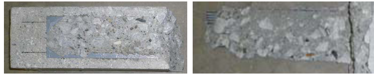
a. failure within concrete substrate (B-1 series)
