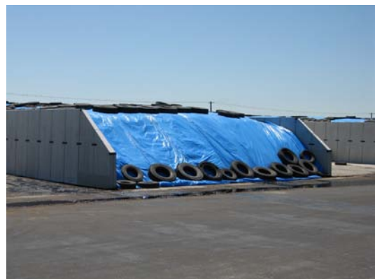
Fig. 4-29. Bunker silo for grass silage covered with polyethylene and used tires.
