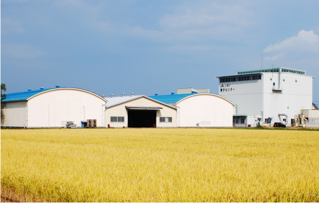
Figure 6. Buildings of Furukawa agricultural cooperative in the Osaki area in the Senpoku Plain.
