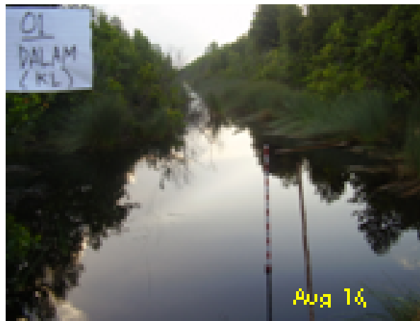
Fig. 74. Tumih after 2 month dam constructed between Dam 02 and Dam 01 at Tanjung canal
