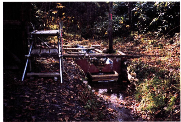
Photo. 3. A dam for measuring water flow.
