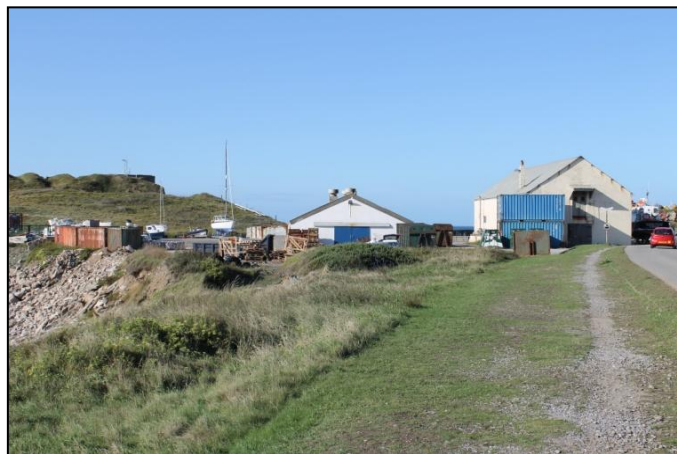
Picture 5-H: View of the recycling centre from the power plant, proposed location for the AD
