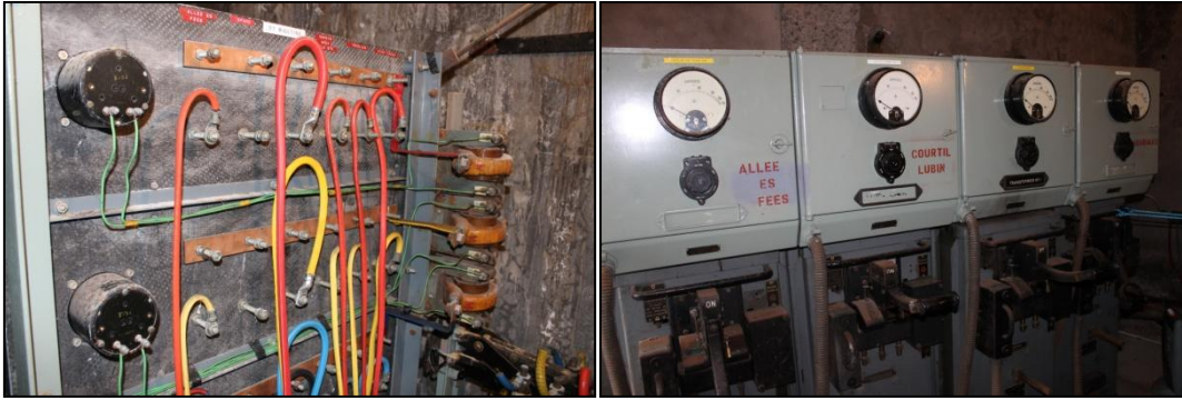
Picture 2-E: Switchgear and main switches of an old substation
