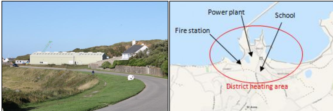
Picture 8-A: View of the power plant from the fire station and map with the possible district heating area
