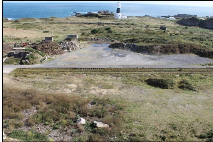
Picture 5-G: Mannez quarry, proposed location for the AD
