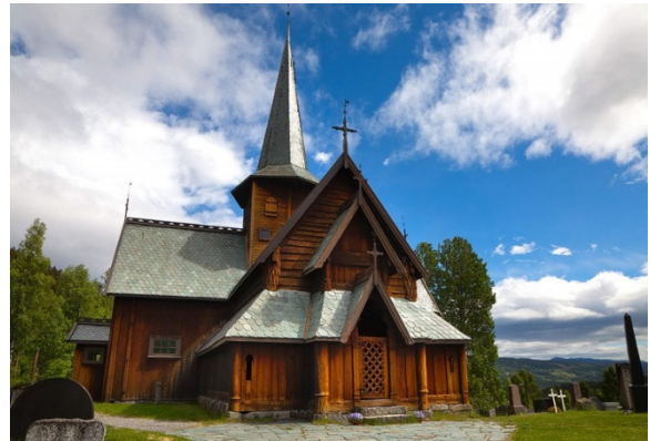
Fig.4.10- Hedalen stave church Fuente: VisitNorway
