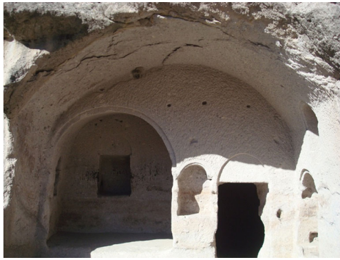
Fig. 11 Spalling of the rock surface in the roof of the room, controlled by rock weathering and stress degradation
