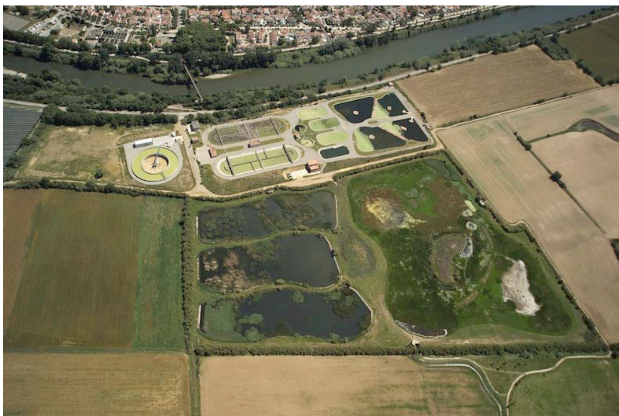
Figure 1.2. Aerial view of the activated sludge WWTP and tertiary treatment constructed wetland system at the Natural Park of Aiguamolls de l'Empordà, Girona, Spain (photo: Consorci Costa Brava).
