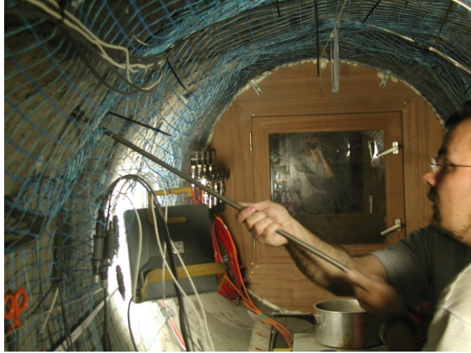
Figure 2: Installation of the instrumentation
