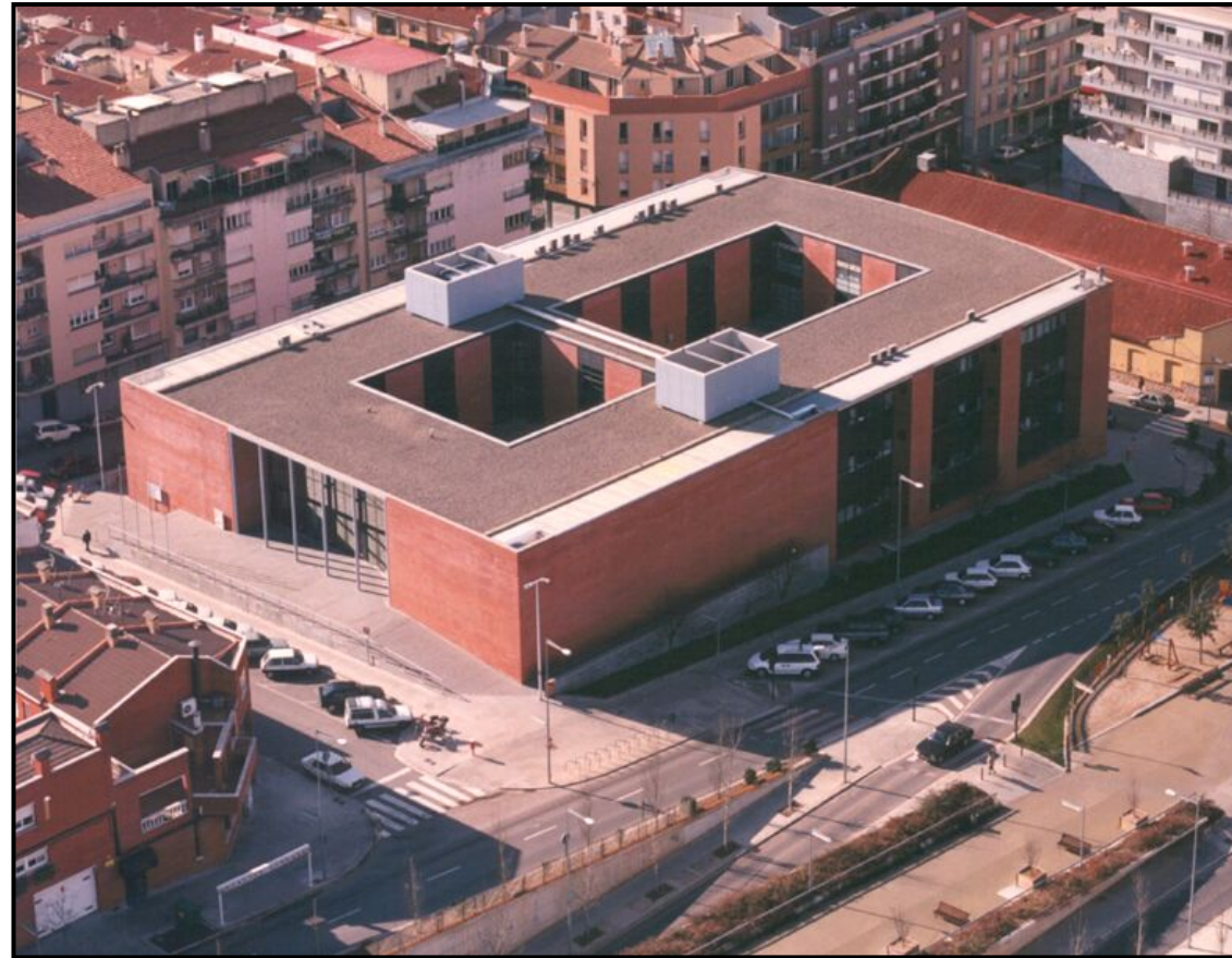
Picture 1: Aerial view
