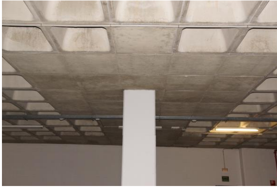
Figure 18: Pillar with two-way flooring
