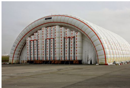
Figure 1.3. Inflatable airplane hangar, BuildAir
