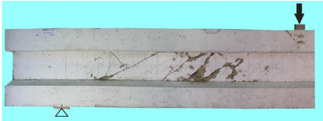
Figure 23: Cracking at failure in experimental S6BN-2.3-12 ( \rho_w = 2.26\% , f_{cm} = 30.7 \text{ N/mm}^2 )(Kurth 2012)
