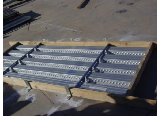
Figure 26 Shoring before concrete pouring.
