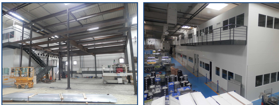
Picture 3.2.6a – Building process of the new module and final results.
