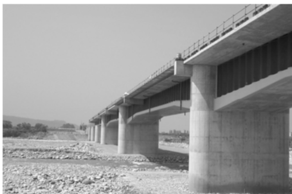
(a) Kurobegawa Bridge
