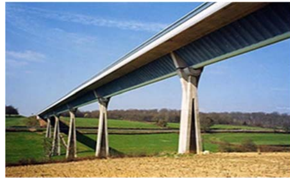
(b) Maupre Bridge
