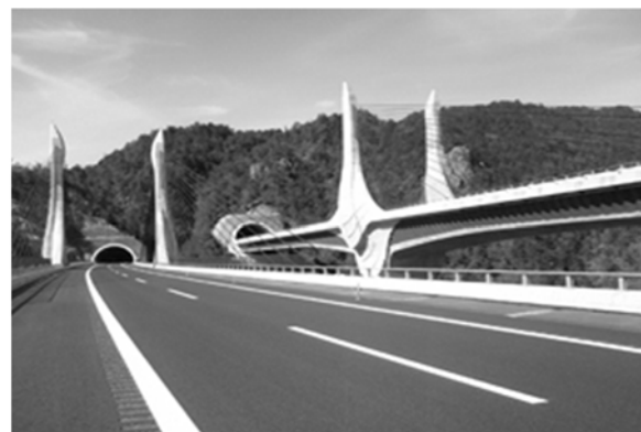
(b) Ohmi-Ohdori bridge
