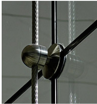
Figure 2.16. Point-fixed clamping device
