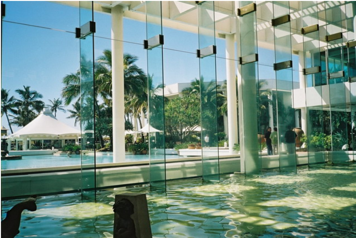
Figure 2.7. Glass fins system; Hotel Sheraton Mirage, Gold Coast, Australia.
