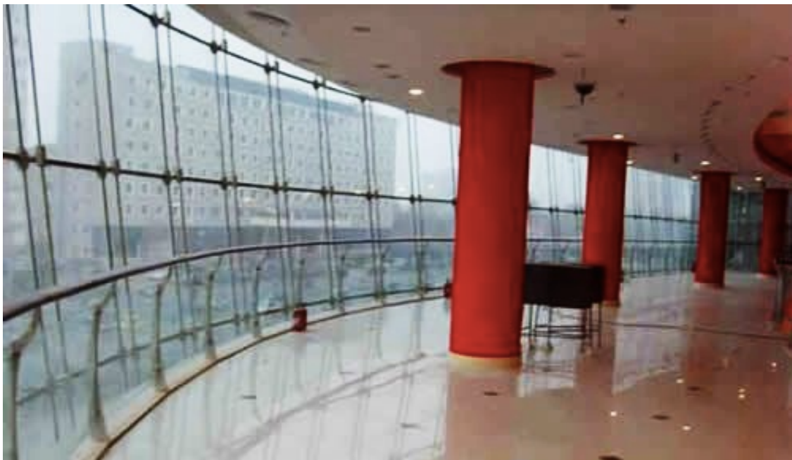
Figure 2.2. One-way cable system; China National Peking Opera Company, Beijing, China.
